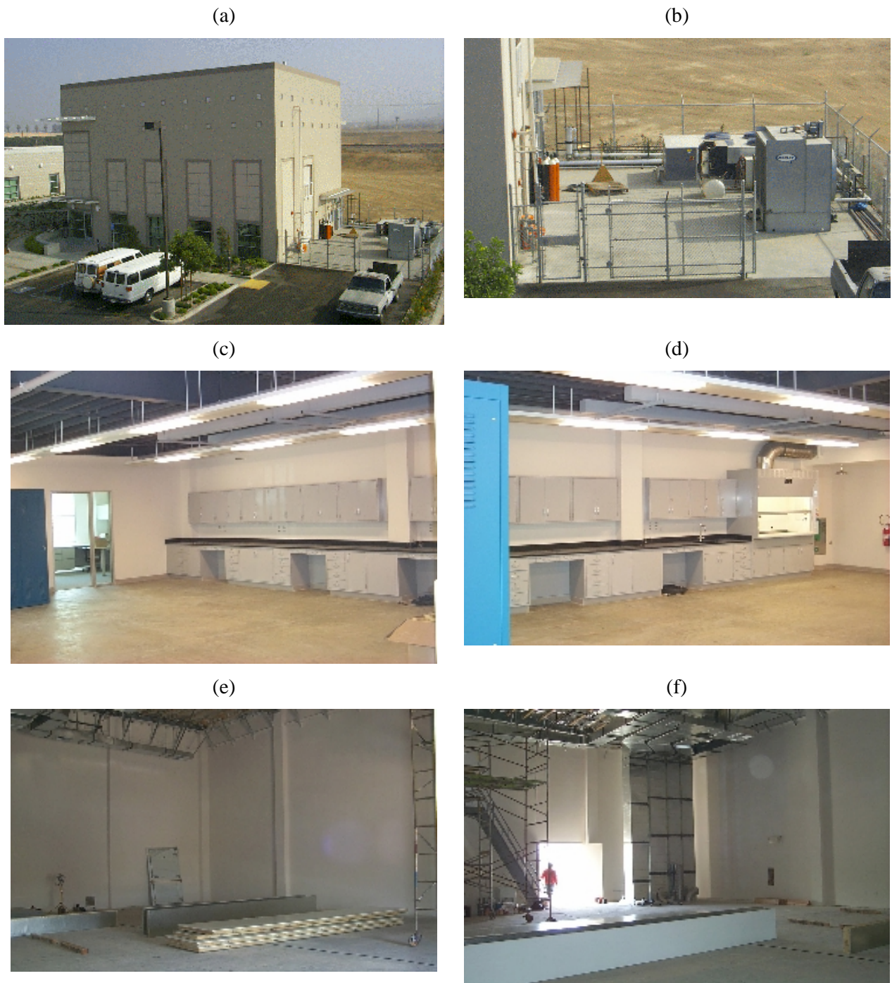
Figure 1. Photographs of the laboratory building constructed to house the new environmental chamber facility. (a) Outside view. (b) Equipment area showing the air purification system and the light and chamber enclosure cooling equipment. (c,d) Laboratory area downstairs. (e,f) Upstairs area during early stages of construction of chamber enclosure.
